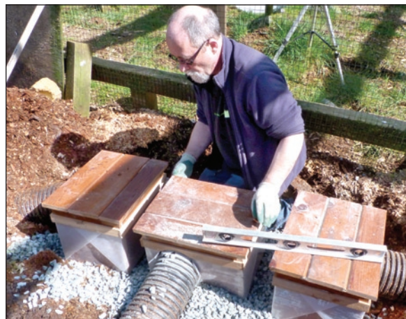
Installation of three new cedar boxes on a bed of drainage rock. — Megan Stuart-Stubbs photo
