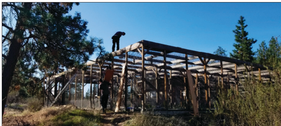
Roof repairs to the Oliver facility. — Lauren Meads photo
