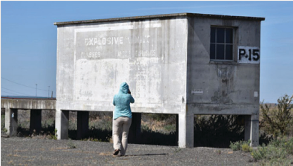
The Umatilla Depot originally had 80 kilometres of interior rail lines. The abandoned train platforms provide homes to ravens, pigeons and occasional song birds. – Adrienne Clay photo
